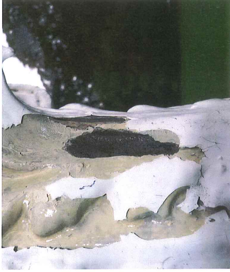
Composite capital paint layers in close up. Evidence of early dark Green layers under cream and white coats. Lead paint (Cream) below Acrylic (White)
